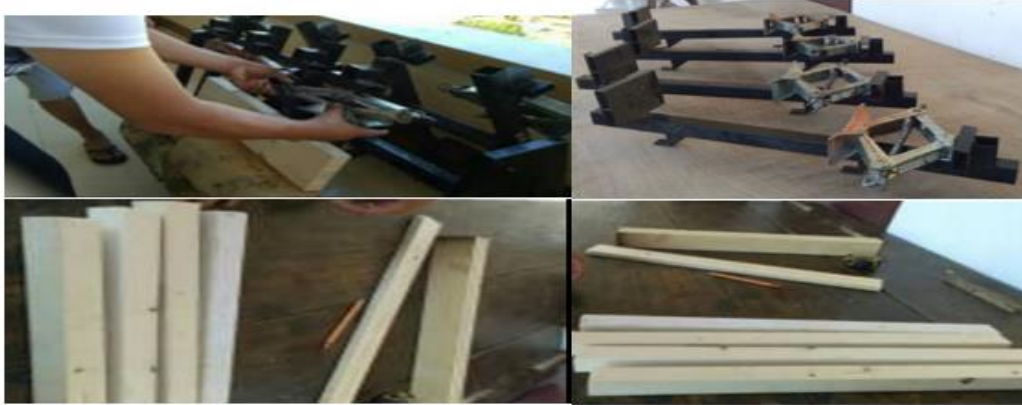
A-Frame Wood Lamination
