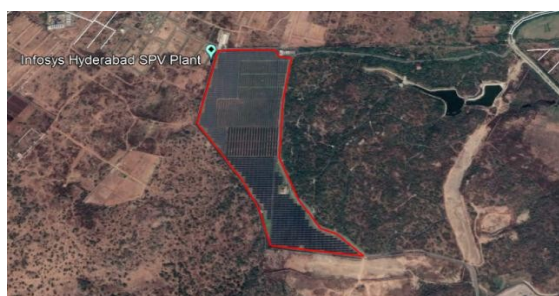
Fig. 3: Geographical location of the Solar PV Plant.
