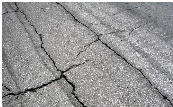
Figure 23 Original of block crack image
