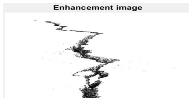
Figure 4 Enhancement of longitudinal crack image
