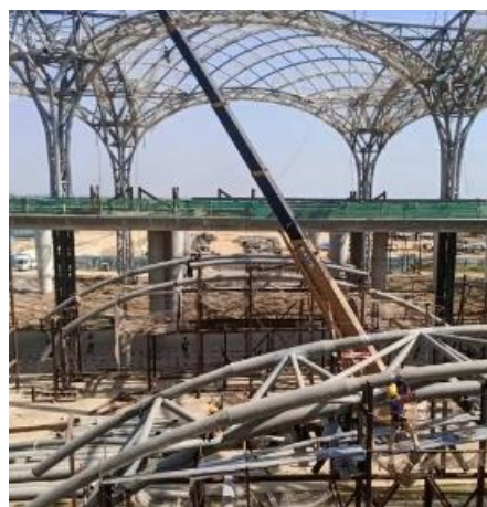
Fig 22 Steel frame lifting on site
