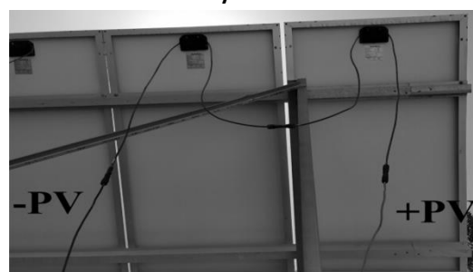
Fig.4.series wiring of two photovoltaic panels
