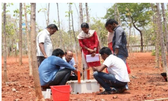
Figure 1: Installation of lysimeter
