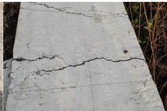
Fig.16. Crack pattern of GPC-GFRP Slab
