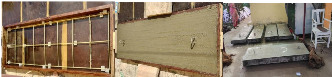
Fig.5. Positioning the reinforcements Fig.6.Casting One way slab Fig.7. Ambient curing of slabs
