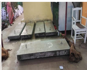
Fig.5. Positioning the reinforcements Fig.6.Casting One way slab Fig.7. Ambient curing of slabs
