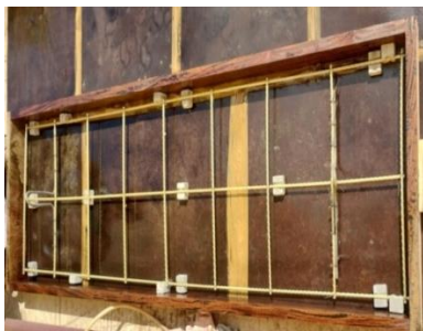
Fig.5. Positioning the reinforcements Fig.6.Casting One way slab Fig.7. Ambient curing of slabs
