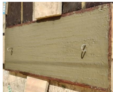
Fig.5. Positioning the reinforcements Fig.6.Casting One way slab Fig.7. Ambient curing of slabs
