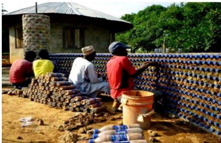
Fig. 8 Wall of eco bricks
