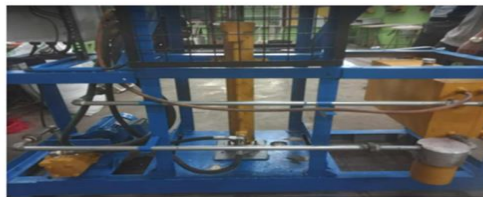
(c) Installation of the hydraulic system components
