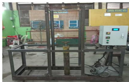
(a) Fabrication of the structural frame
