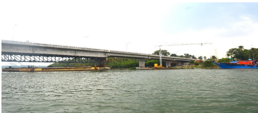
Fig 7: Aravila Bridge, Parakkadavu, Kollam, Kerala (Buoy Number 301-302)
