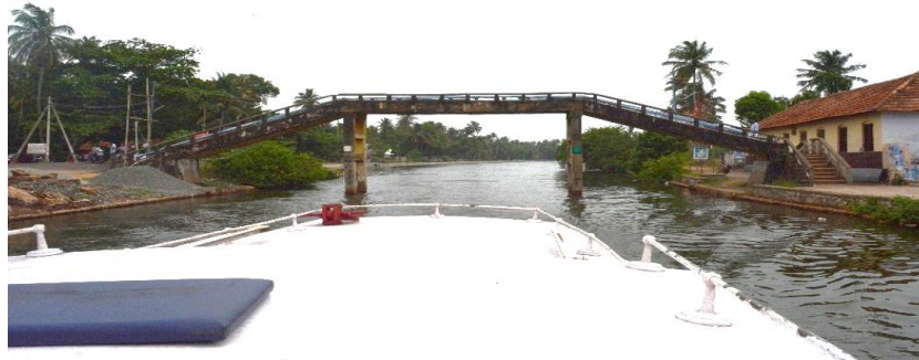
Fig 8: Kovilthottam Bridge Chavara, Kerala (Buoy Number 294-295)
