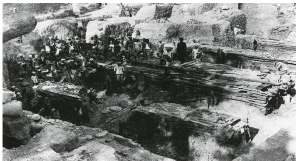
Fig 8: Wooden platforms just south of the hall, thought to have supported a staircase to the canal (Spooner D. B., 1912-1913).
