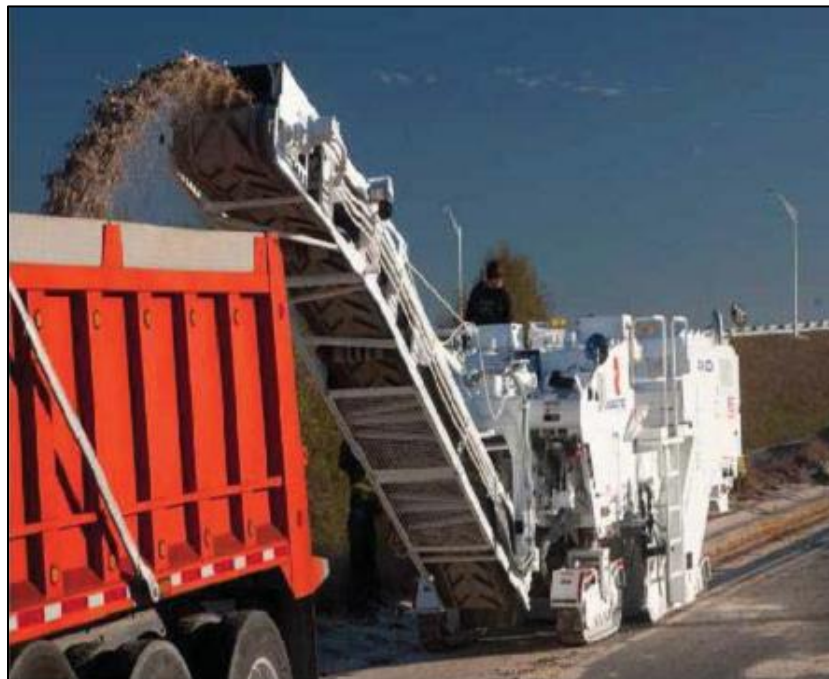
Figure (4): Milling of Asphalt Pavements [40]
